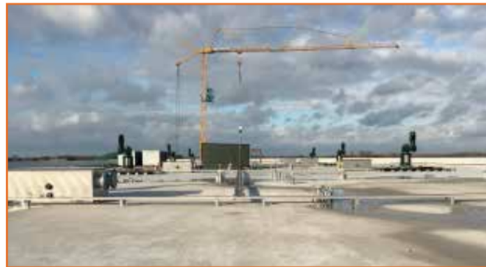
Overview of the top of the tank
